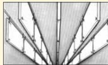
Absorbers can be hung in parallel rows two feet apart, or in an egg-crate configuration.
